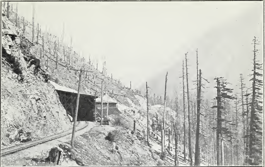
FIG. 1.—THE WELLINGTON AVALANCHE, WHICH KILLED 100 PERSONS, OCCURRED ON THIS SLOPE, THE FOREST ON WHICH HAD BEEN DESTROYED BY FIRE.
